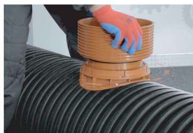
11. Setting the selected connection
