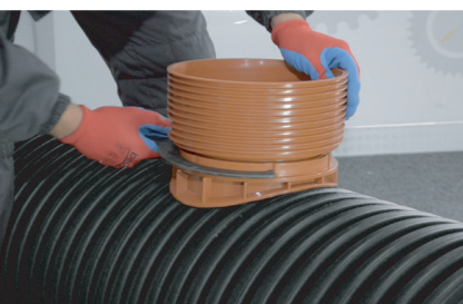
12. Final tightening of sag
