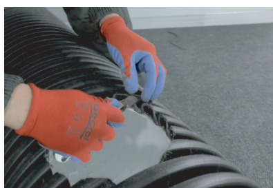
5. Cleaning chips and forming a clear hole
