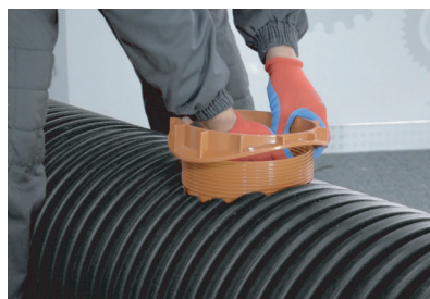
8. setting the spacer ring
