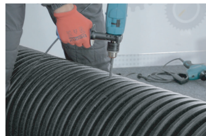
3. Drilling holes for the guided crown saw
