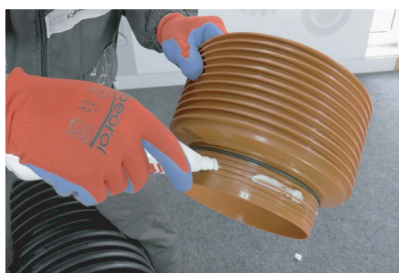
10. Lubricating appropriate connection of sag
