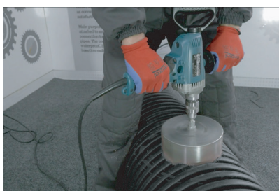
4. Drilling holes with crown saw
