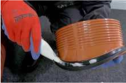
6. Lubricating rubber bands on the body of sag
