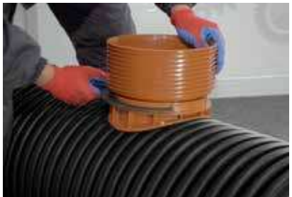
12. Final tightening of sag
