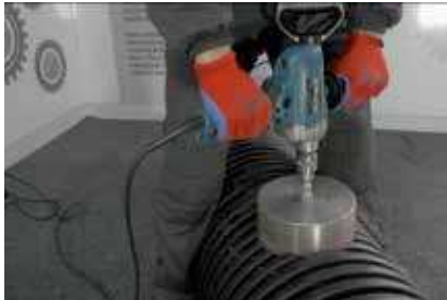
4. Drilling holes with crown saw
