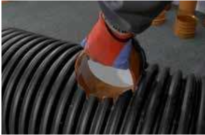
7. Inserting body of sag through pre-prepared opening and setting int in the appropriate position
