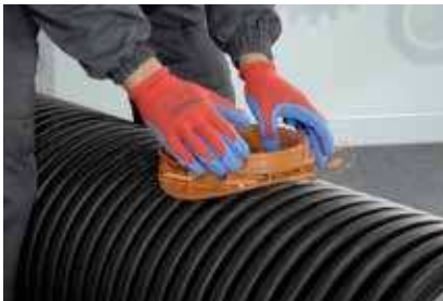
9. Tightening the sag
