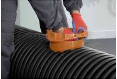
8. setting the spacer ring
