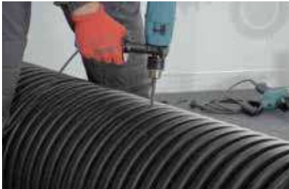
3. Drilling holes for the guided crown saw
