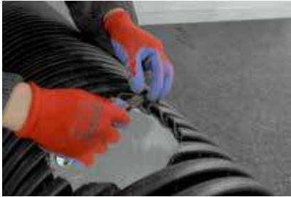
5. Cleaning chips and forming a clear hole
