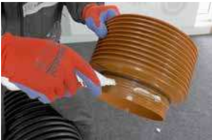
10. Lubricating appropriate connection of sag
