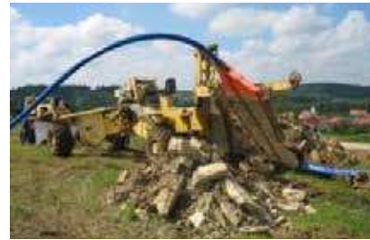
Installation without digging an open trench, method of pipe laying - ploughing.
