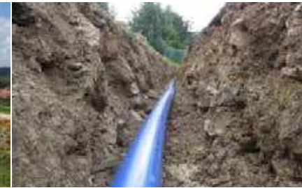
Installation without sand bedding
