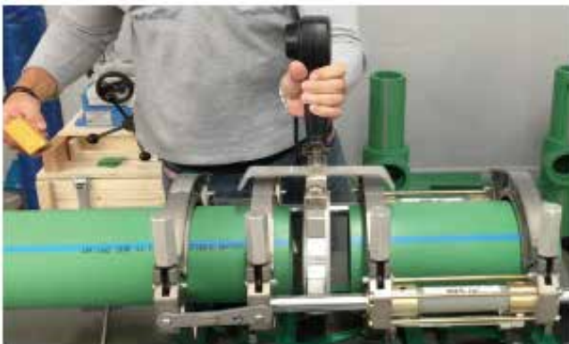
Picture no. 43: Insertion of the heating plate
