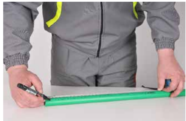
Picture no. 21: Marking the required depth of cheeses. The required welding depths along pipe diameters can be taken from the following table:
