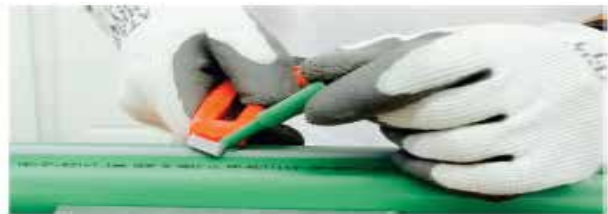
Picture no. 49: Cutting off of the reparation plug
