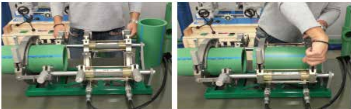
Picture no. 41: Fixing the pipe with jaws
