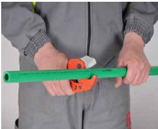
Picture no. 19: Cutting PP-R and PP-RCT pipes
