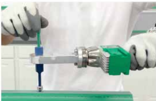
Picture no. 47: Inserting reparation tools
