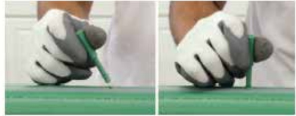
Picture no. 48: Inserting the repacking plug
