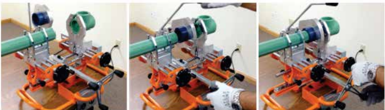
Picture no. 38: The installation of pipes and fittings in the teflon head
