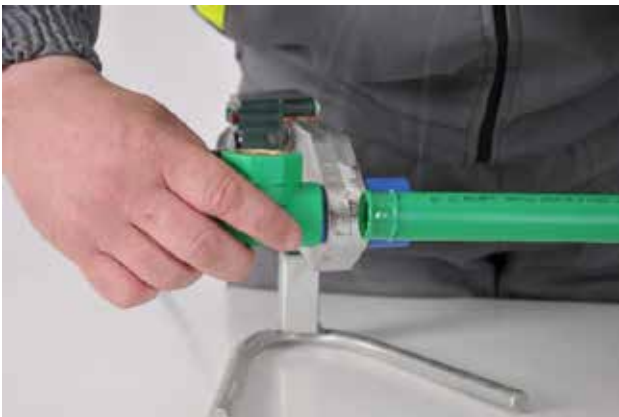
Picture no. 24: Connecting the pipe with the fitting
