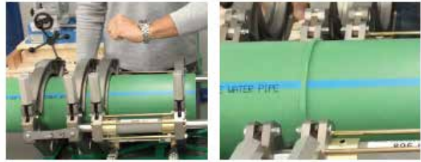
Picture no. 44: Butt Welding
