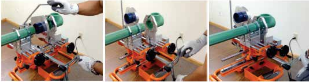
Picture no. 39: Welding and cooling of pipes and fittings
