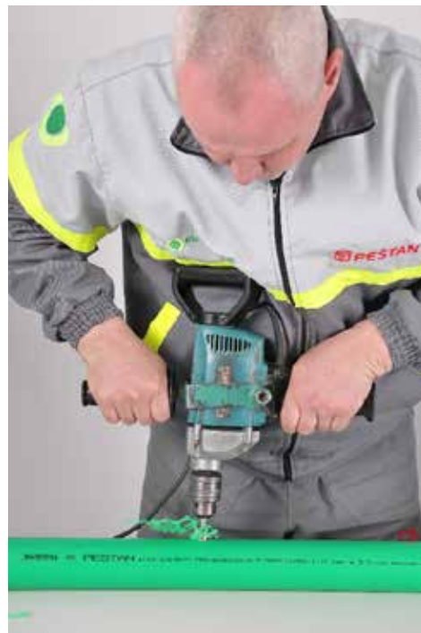
Picture no. 27: A method of drilling pipe
