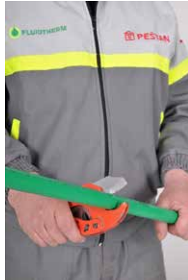
Picture no. 33: Displays the cutting of the pipe with scissors
