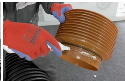
10. Lubricating appropriate connection of sag
