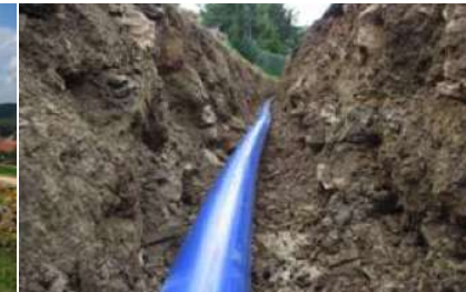
Installation without sand bedding
