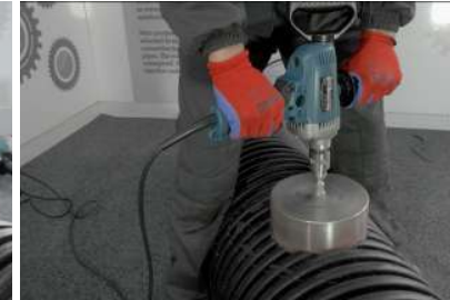
4. Drilling holes with crown saw
