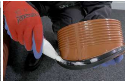
6. Lubricating rubber bands on the body of sag
