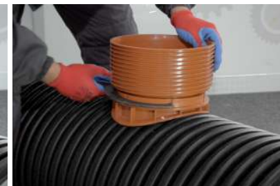
12. Final tightening of sag
