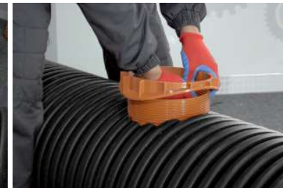
8. setting the spacer ring
