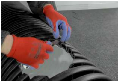
5. Cleaning chips and forming a clear hole
