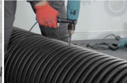
3. Drilling holes for the guided crown saw
